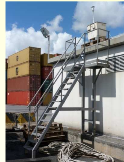
TERMINAL RAVANO (Skypost ARPAL)
